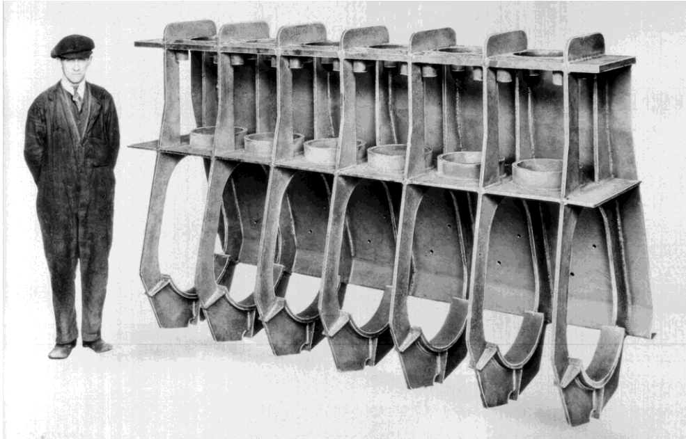
Figure 6. Stevens' patent welded steel engine frame.
